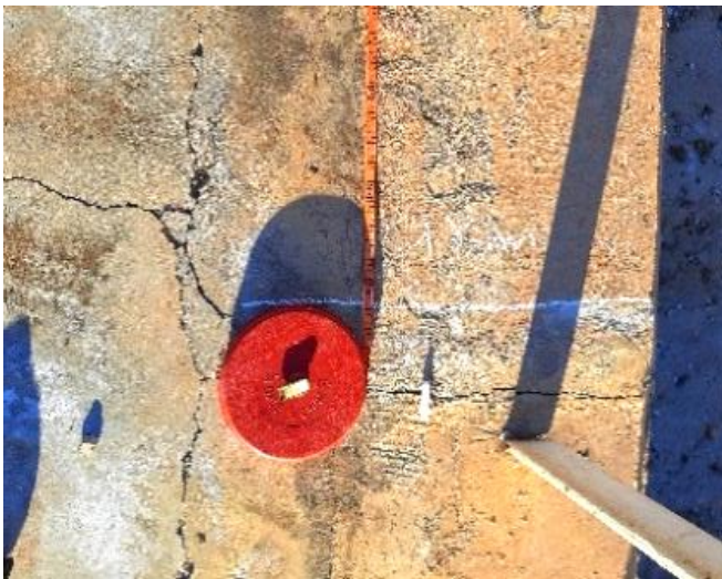
Fig. 6 Measurement of span length
