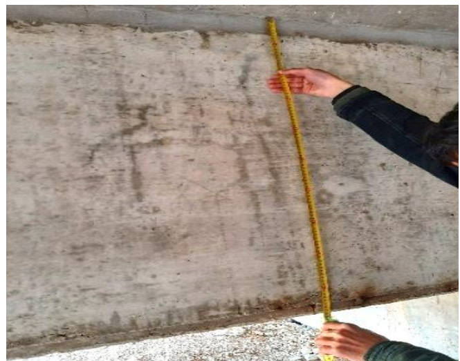
Fig. 9 Measurement of the beam's flange height
