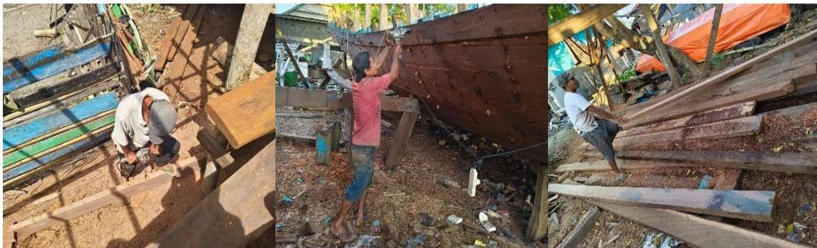
Fig. 3 Material and construction of a traditional shipyard
