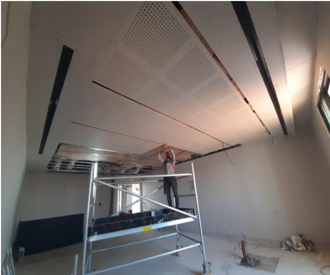
Fig. 4 Suspended ceiling
